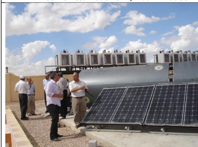
Innovative Renewable Energy (RE) Driven - Multi Stage Flash (MSF) System with Salts Precipitator and Nano Filtration (NF) Feed Water pre Treatment (RE-NF-MSF). (Faculty of Agriculture, Alexandria University)
