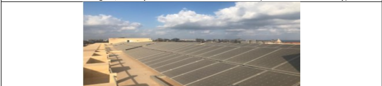
Solar photovoltaic with a capacity of 220 kilowatts on the 2000 m 2 roof top of the building of the Mechanical Engineering Department at the Faculty of Engineering
