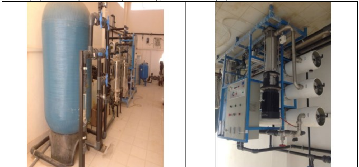
100 m3 Desalination Unit, Wadi El-Natroon (Faculty of Agriculture, Alexandria University)
